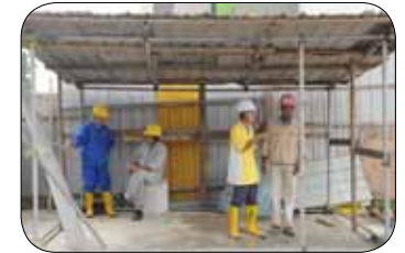
Figure 6.3: Workers' rest point under shade. †
