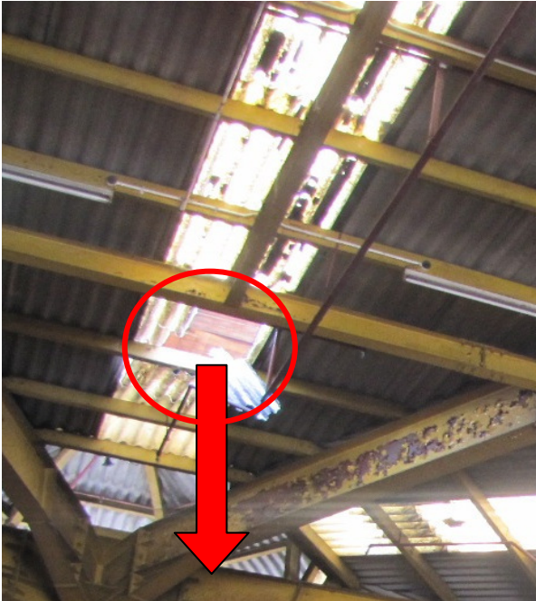
Fragile roof skylight where a worker stepped on and fell through in a fatal accident
