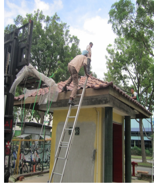
Work on roof
